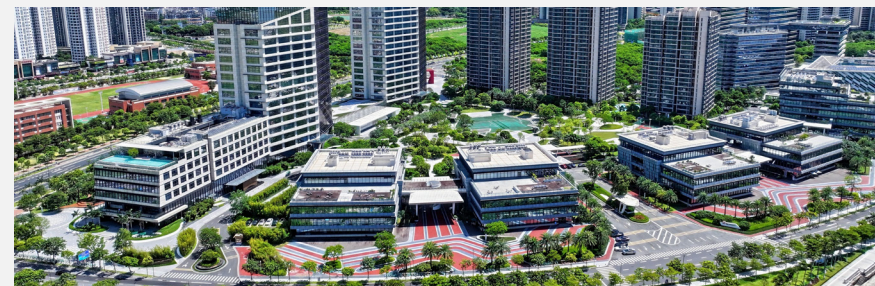
The R&D Zone Phase II of Zhuhai Kingsoft Campus
